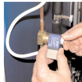
Montage de la bobine Mounting of the coil Montage der Spule
